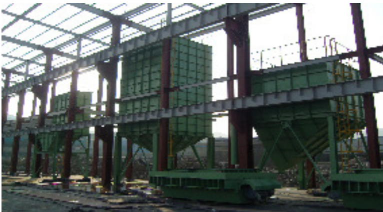
Dust collectors: • 1×400m 3 /min, • 2×600m 3 /min, • 2×1000m 3 /min
